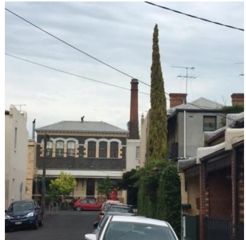
The chimney is west from the western boundary of 40 Bell St, and west from the eastern boundary of 45 Moor St.
